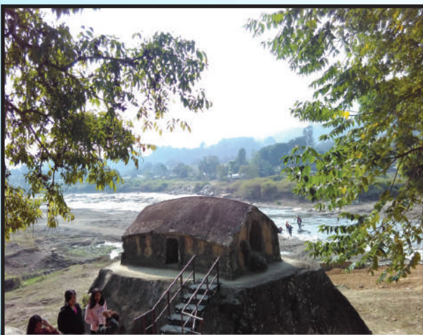
Image 1: Showing the Stone house situated beside the river, Mahur in Maibang, Dima Hasao (source- Author).
